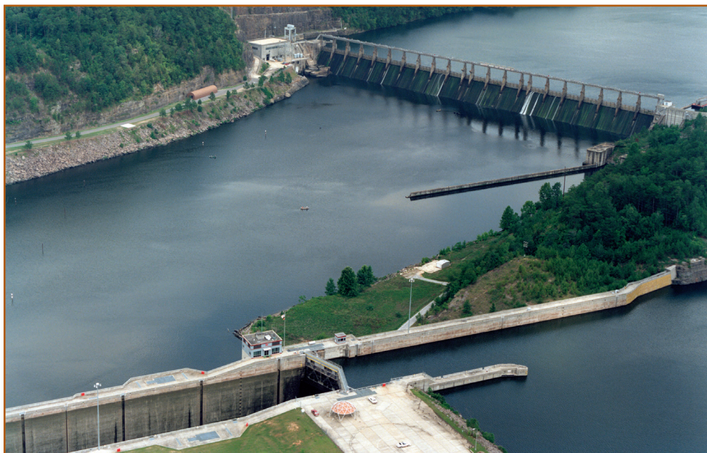
The redeveloped Bankhead Lock and Dam. One wall of the old lock remains near the dam. The powerhouse went into operation on July 12, 1963.
