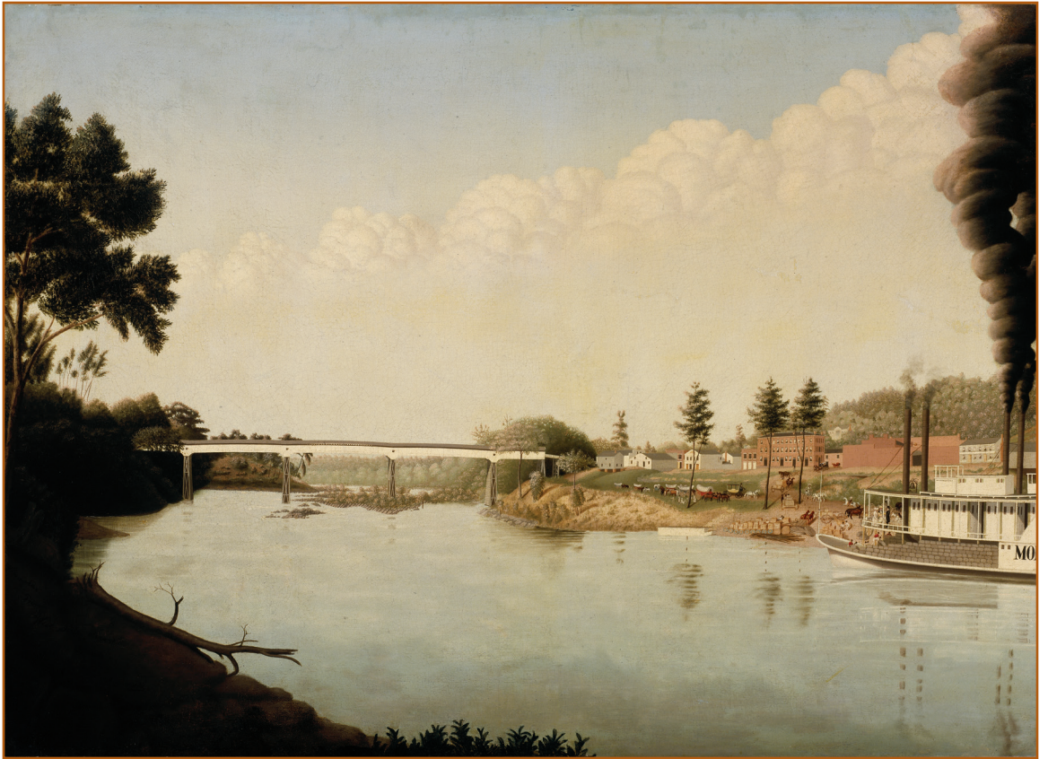
Shoals on the Coosa prevented river traffic north of Wetumpka. Wetumpka Bridge, Adrian E. Thompson, 1847. Courtesy of the Museum of Fine Arts, Boston.
