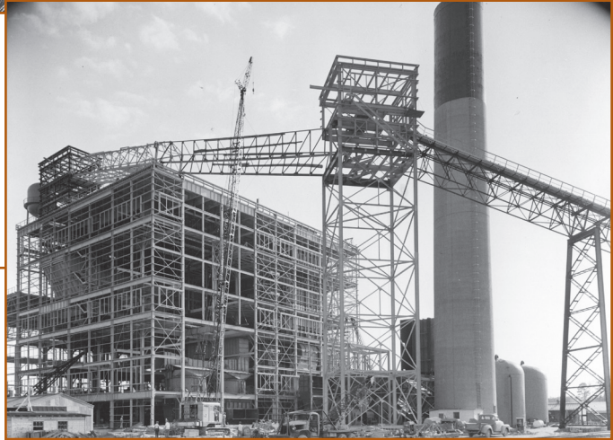
Barry Steam Plant under construction, October 5, 1953.
