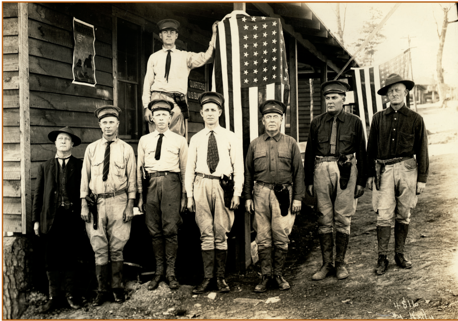
Federal marshals stationed at the Warrior Reserve plant during World War I while unit No. 2 was under construction.
