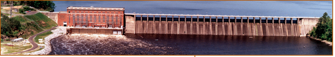
Downstream view of Lay Dam showing the redevelopment completed in February 1967.
