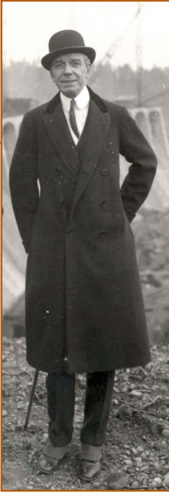
Sir E. Mackay Edgar at a visit to the Jordan Dam site, February 15, 1928.
