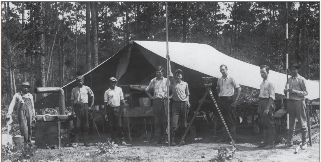
Transmission line survey crew, Lock 12 line, September 16, 1913.
