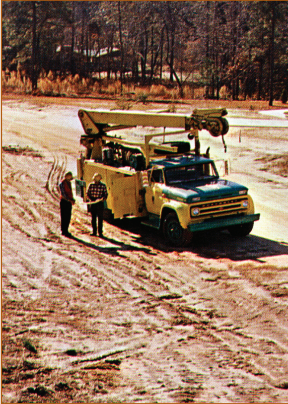
Bucket trucks revolutionized line repairs.
