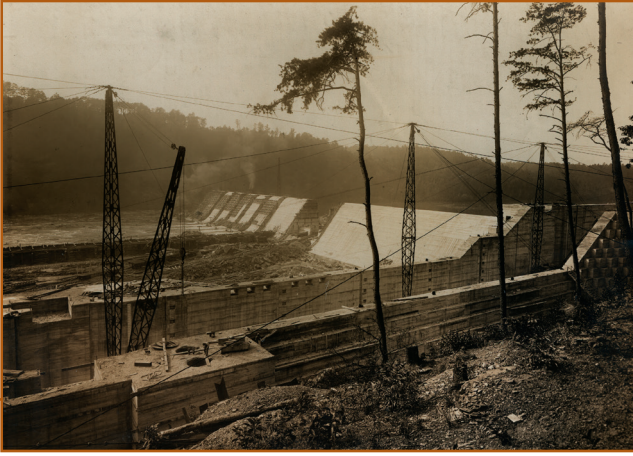
U. S. Army Corps of Engineers Lock 17 project on the Warrior River, May 22, 1914.
