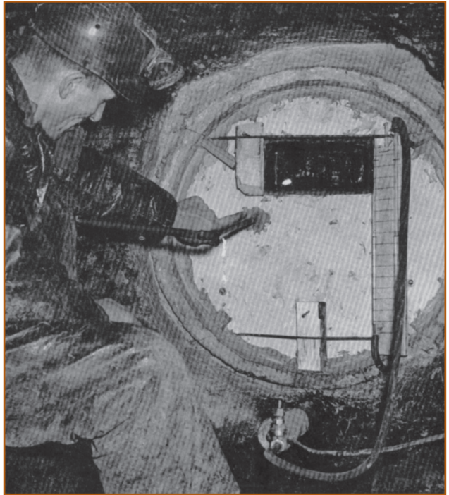
Tom Boykin of Gorgas mines seals up crevices in one of the coal gasification access holes before firing.
