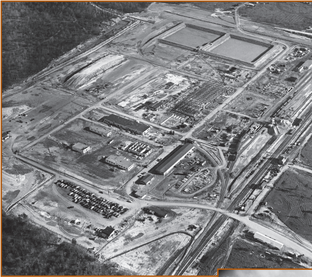
Olin Matheson Chemical Company under construction, ca. 1952.
