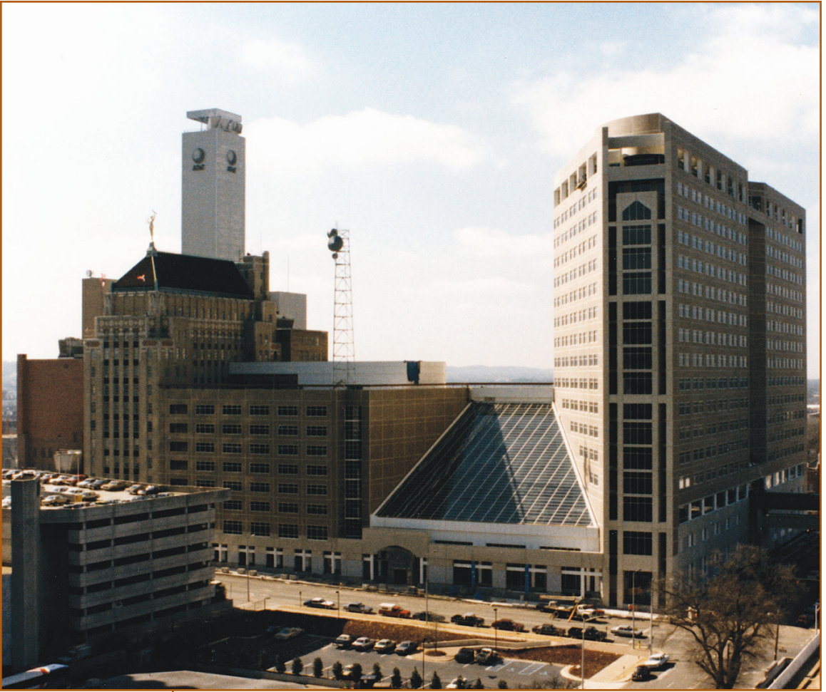
Alabama Power Company's corporate headquarters under construction. An atrium connected the new north tower, completed in 1986, with the south tower and the original 1925 art deco building.
