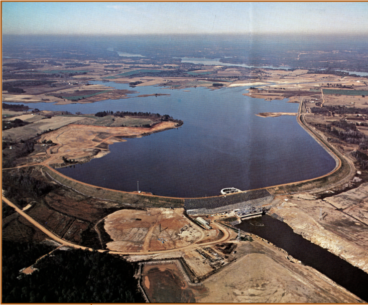
Bouldin Dam has the largest generating capacity of all Alabama Power's hydroelectric plants.
